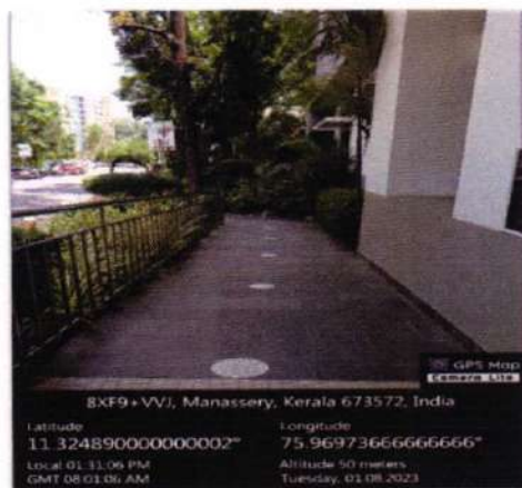
RAMP IN FRONT OF COLLEGE
